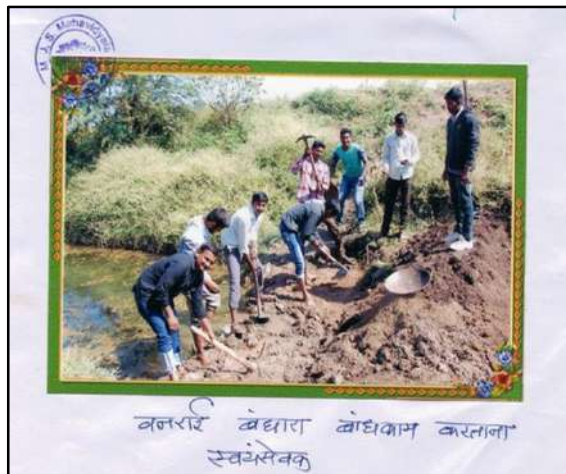
Trench digging for bandhara construction.
